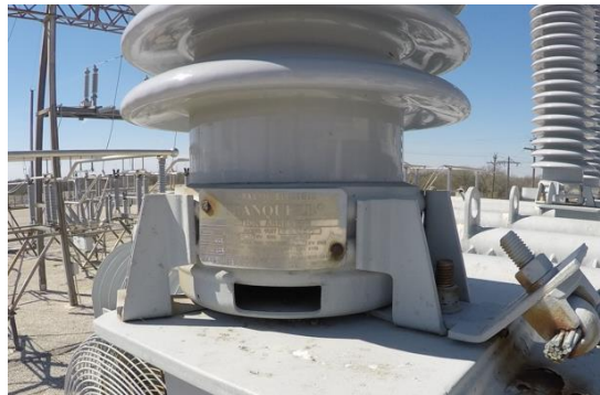
Replaced Nine 39-year-old Surge Arresters Figure 5
