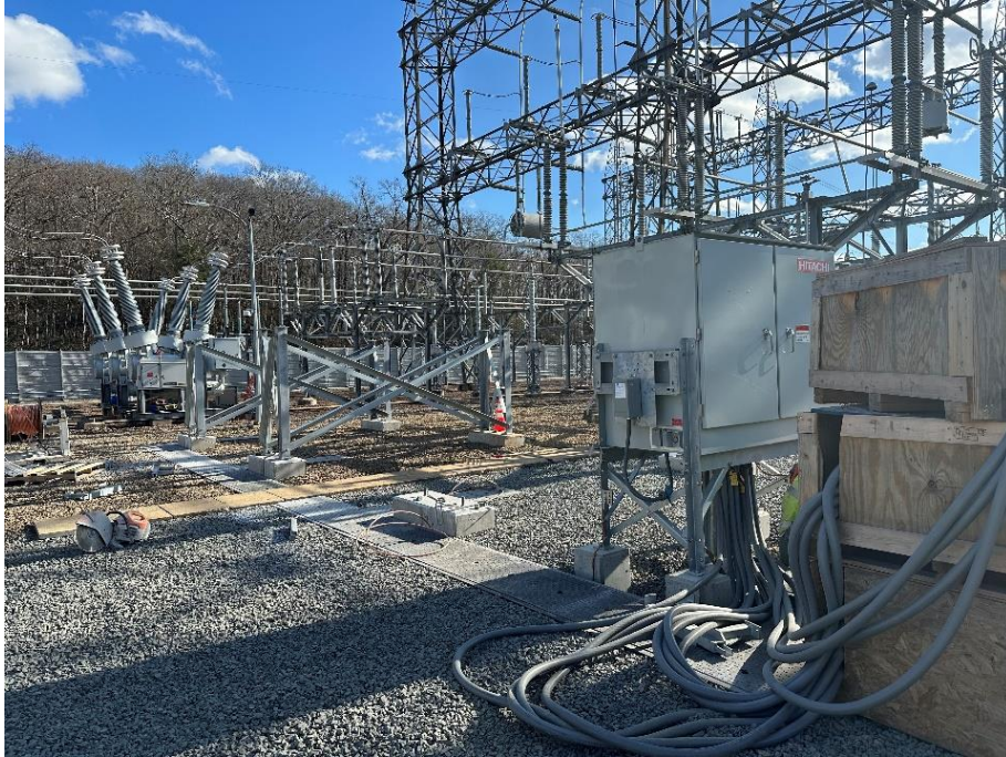
Preparation of Interphase Cabling Figure 7
