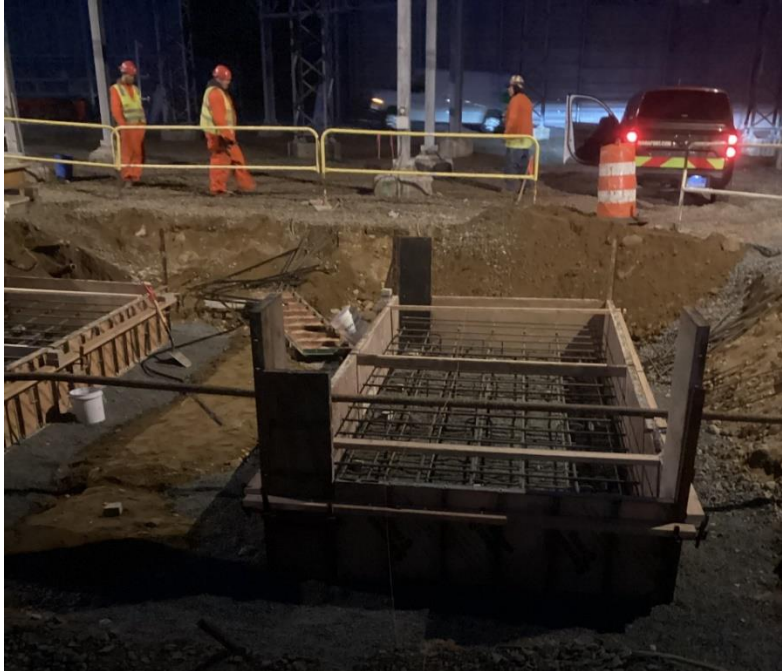
Site Preparation for New Concrete Footings Figure 5
