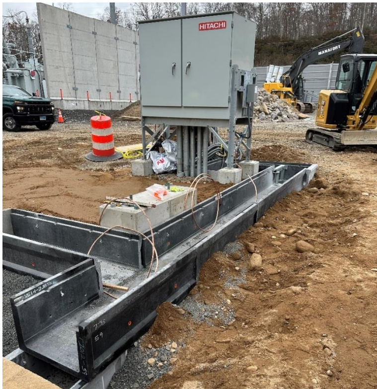
Installation of New Cable Raceway Figure 6
