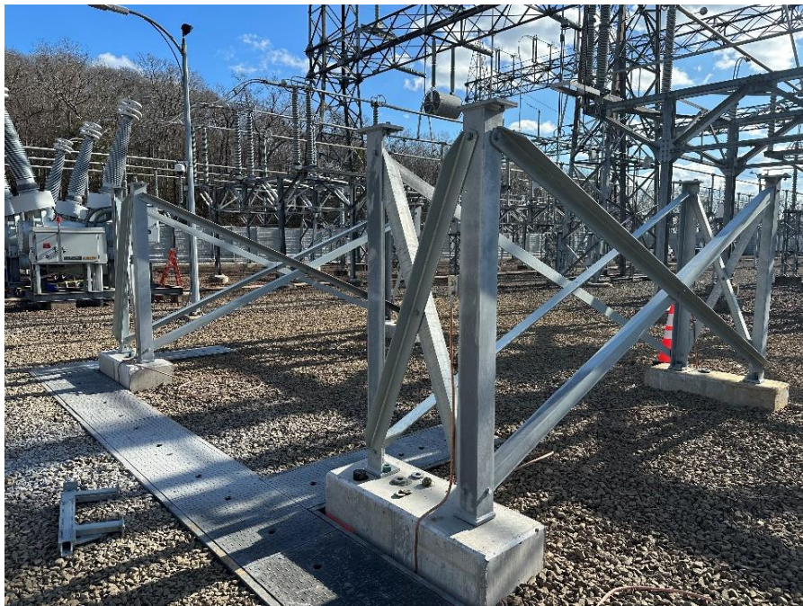
Erection of New Breaker Frames Figure 8
