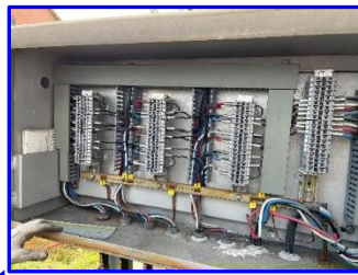
a) Junction box at CT side where W, X and Z are grounded
